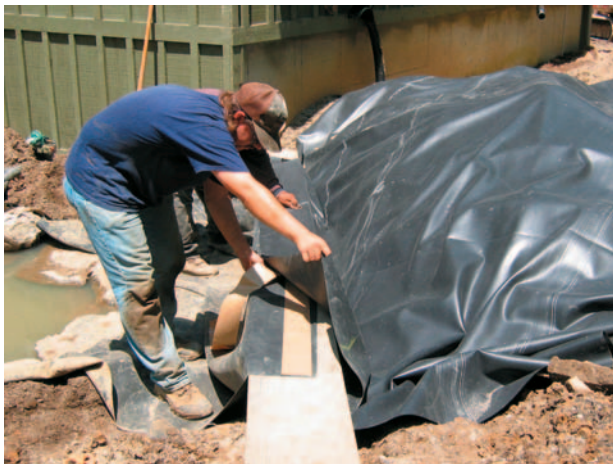
Gently peel the tape paper while applying pressure to bond the top piece of liner.
