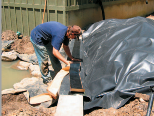
Once again clean the entire surface of the liner and apply the cover tape.
