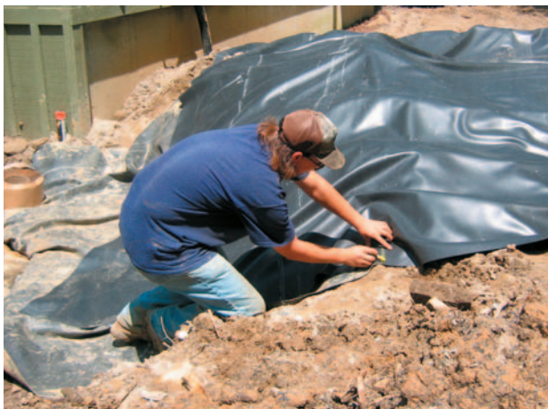
Overlay the top piece to match the bottom piece and mark both ends where the seam will be.
