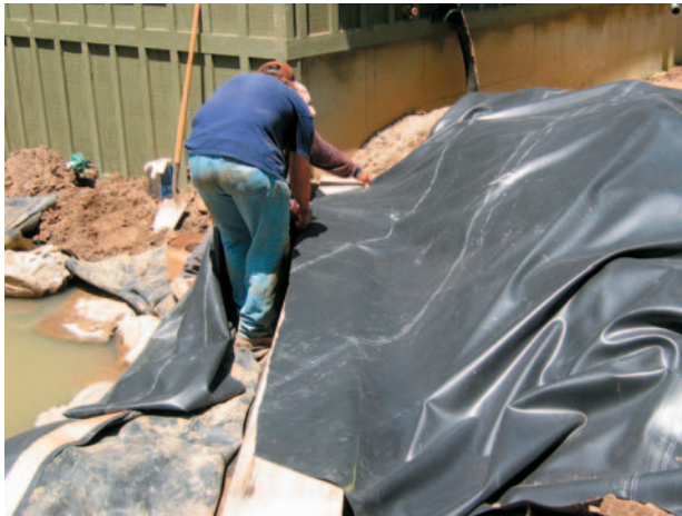
Lay the top piece over the bottom piece matching the alignment hash marks. Trim any excess using the 2"x12" as a straight-line guide.
