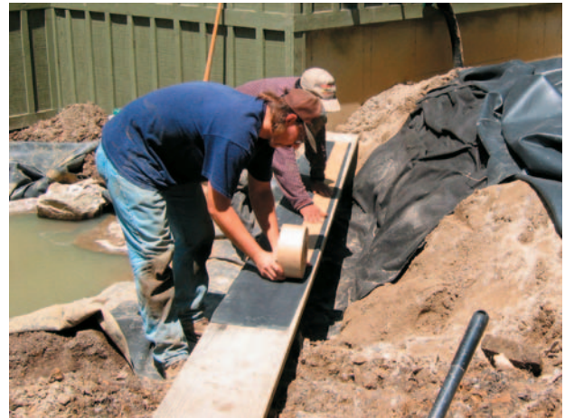
Using the edge of the 2"x12" for a straight edge guide, apply the 2-sided tape and trim excess liner.
